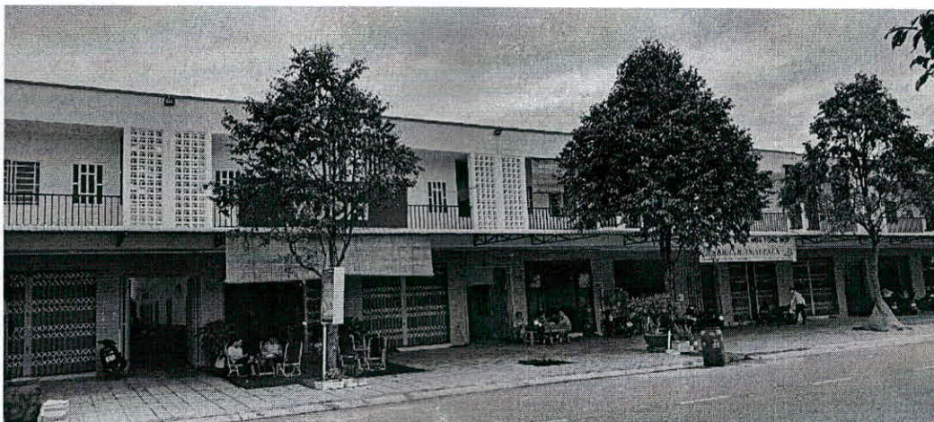
House picture at Plot A51/Bau Bang (Transferred to customers)
