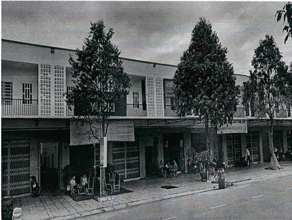
House picture at Plot A51/Bau Bang (Transferred to customers)
