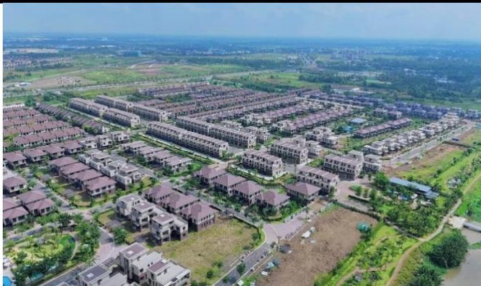
Hình 25: Waterpoint – GD 1 (Southgate); Waterpoint – GD 2 (VCD)
